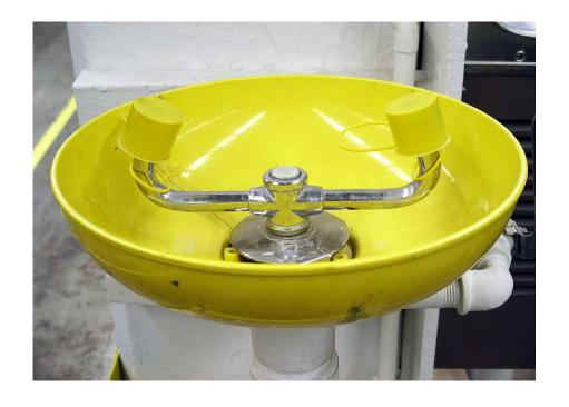
Equipment that flushes the eyes and face with water to remove chemicals, debris or irritants
